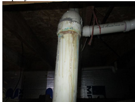
Moisture stains in basement
