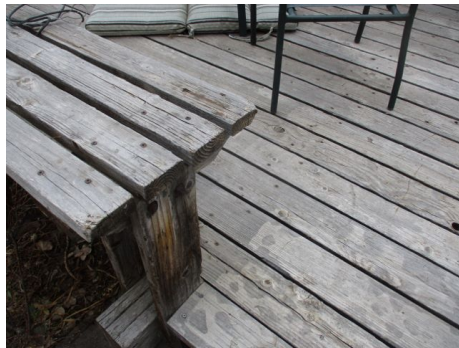
Weathering on decks
