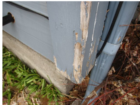
Weathered wood & peeling paint on windows & trim
