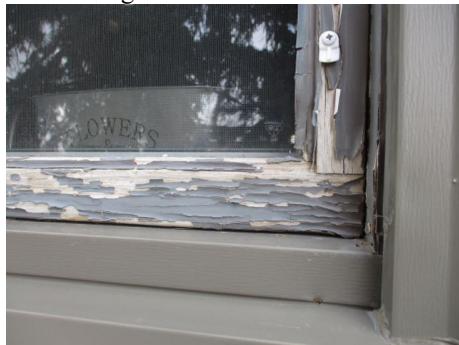
Weathered wood & peeling paint on windows & trim
