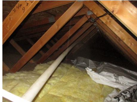
Improper slope on plumbing vents in attic
